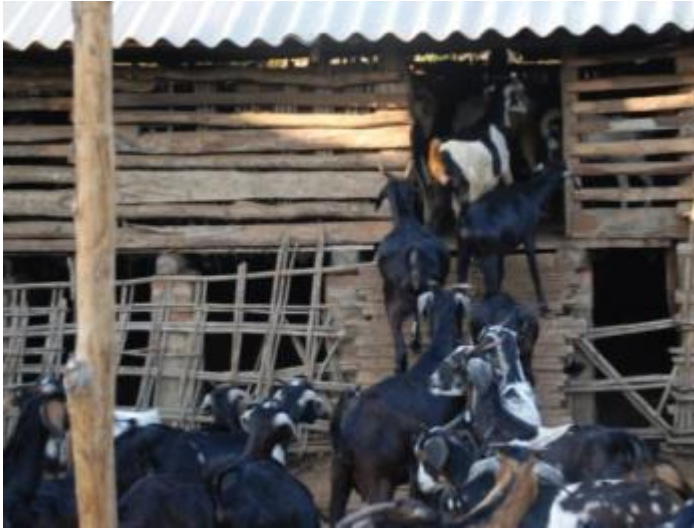
Upper storey goat shed manure accumulates below
